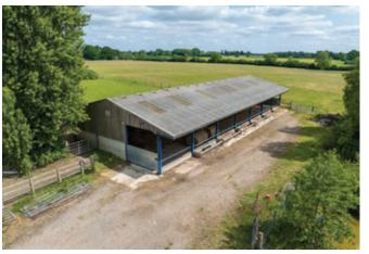
A canopy, formed as part of the steel frame runs along the entire principal elevation. The floor is constructed from a 190mm concrete ground bearing floor slab. The building is in good overall condition.
